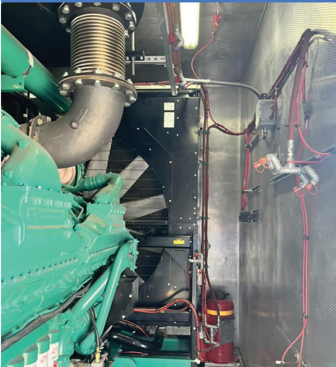
In just 3 days time the on-site technicians at BGR Radiator completed this 60L Cummins Generator radiator core replacement.
