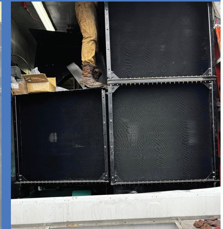
In just 3 days time the on-site technicians at BGR Radiator completed this 60L Cummins Generator radiator core replacement.
