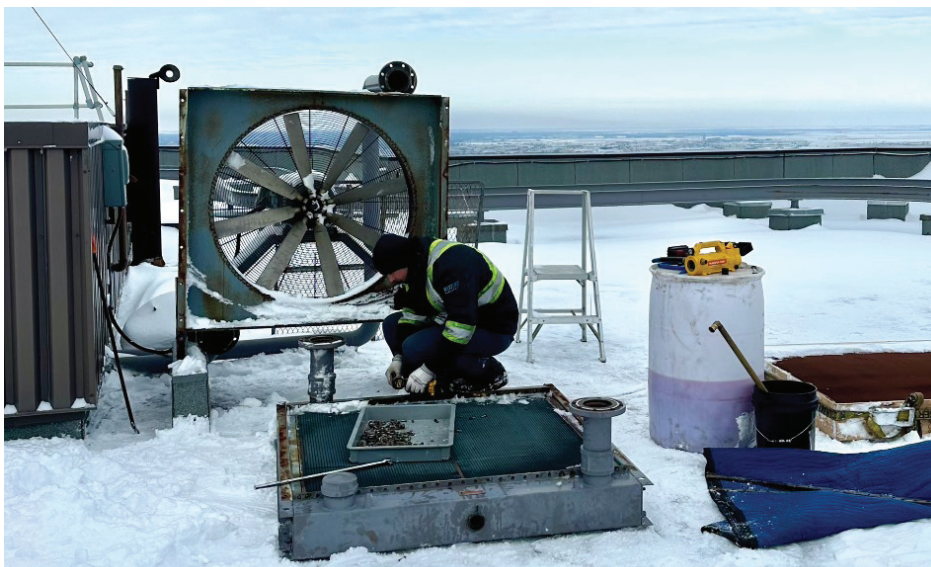
Check out these rooftop views from a recent backup generator job the team at West End Radiators did for a building in downtown Winnipeg. Their mechanics recored the radiator with a higher-efficiency brass core that will be able to withstand the high winds and cold temps it sees on this rooftop.
