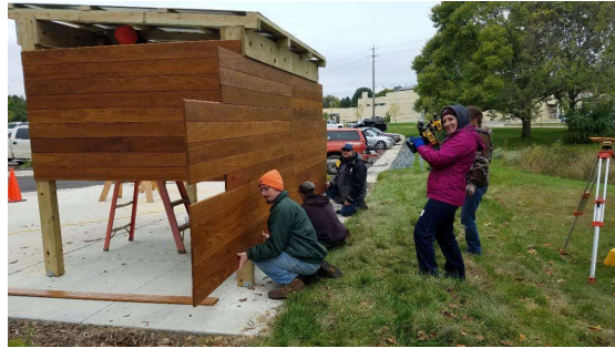
Ash wood, green roofed bike parking at the Heintz Center, RCTC, Rochester, MN. Credit: Angela Gupta, UMN Extension
